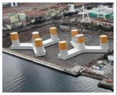
semi-sub-type Hybrid floating structure
